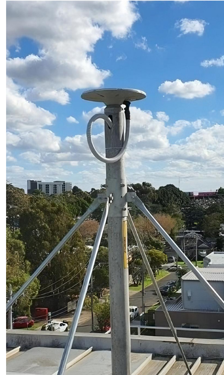
Source: GPSnet GNSS reference station in Heidelberg to support North East Link
